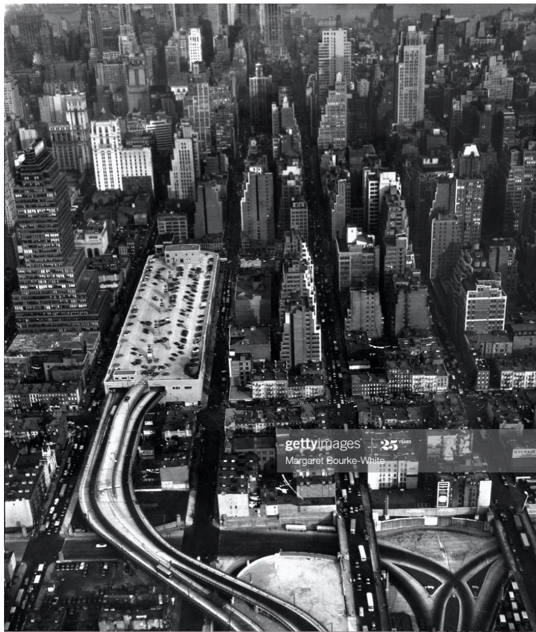
Lincoln Tunnel Ramps, PA Bus Terminal (1951, Getty Images)
